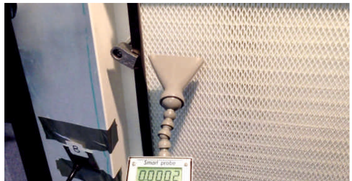
HEPA LEAK SCAN TEST
