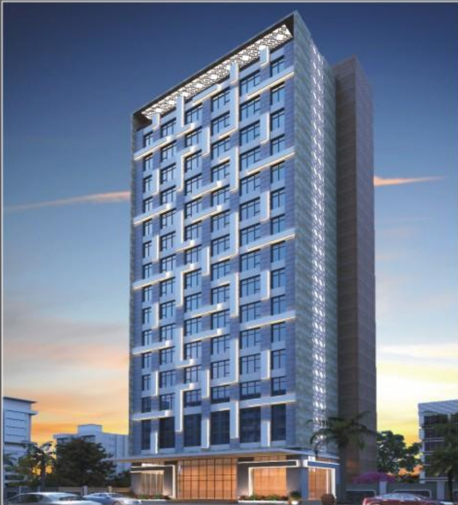
Oshiwara Hotel, Mumbai Area : 72,000 sq ft , MEP Cost :86,400,000
