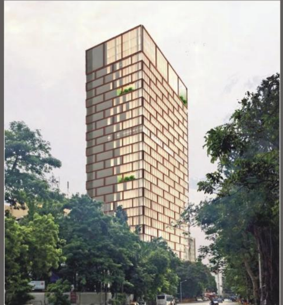
Essel Continental, Worli, Mumbai (LEED Gold Rating) Area : 500,000 sq ft , MEP : 625,000,000
