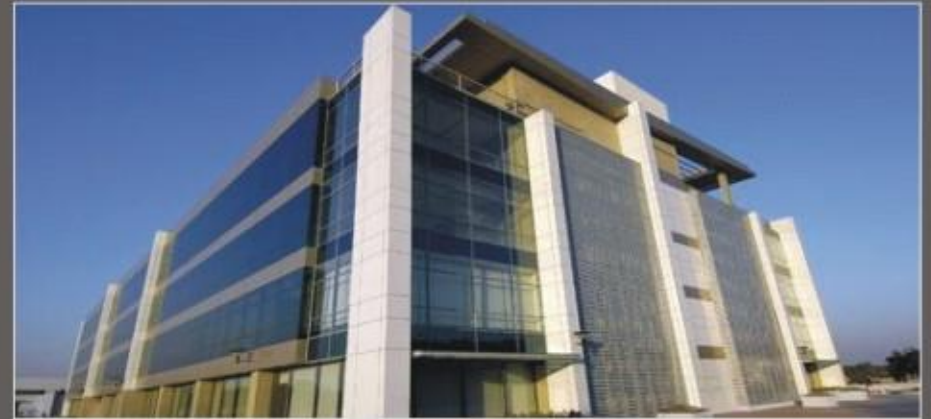
JOHN DEERE OFFICE, PUNE AREA : 200000 sq ft , HVAC : 475 TR
