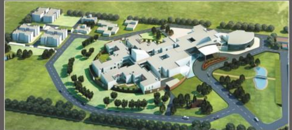
NIREH, Bhopal (LEED Gold Rating) Area: 150,000 ft 2 , HVAC Cost : Rs. 80,000,000
