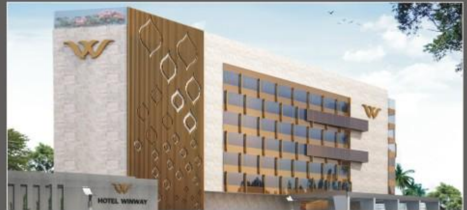
WOW Hotel, Indore (ECBC Compliant) Area: 250,000 ft 2 , MEP Cost: Rs. 150,000,000
