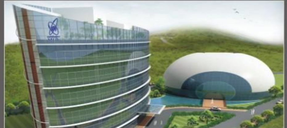
RAPP, Kota, Rajasthan Area: 65,000 sq ft , MEP Cost: 59,000,000
