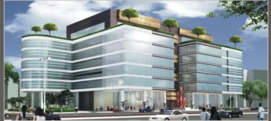
Satellite Gazebo,Andheri,Mumbai Area: 2,50,000sq ft , HVAC Cost Rs. 90,000,000
