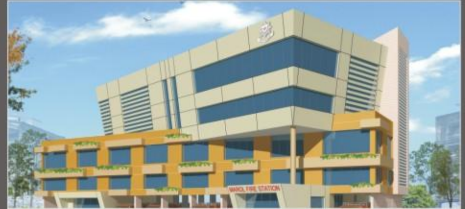
Marol Fire Station, Mumbai
