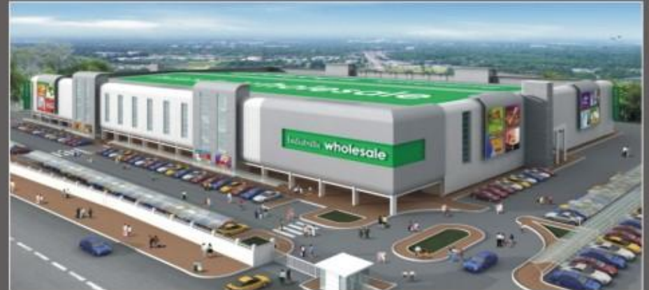
INDIA BULLS WHOLESALER, AHMEDABAD AREA:270000 SQ. FT. ;HVAC:1400 TR
