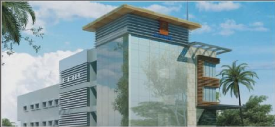
Kongsberg Corporate Office Navi Mumbai Area: 25,000 sq ft, HVAC Cost : 5,400,000
