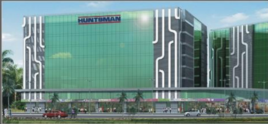
Huntsman R&D Center, Mumbai Area: 250,000 ft 2 , HVAC Cost: Rs. 90,000,000
