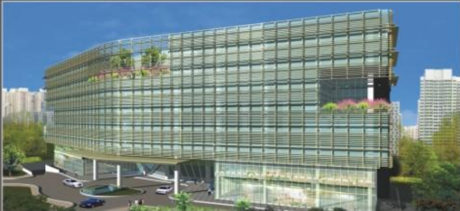
Satellite S-14,Andheri,Mumbai Area : 2,50,000 sq ft , HVAC Cost Rs. 90,000,000
