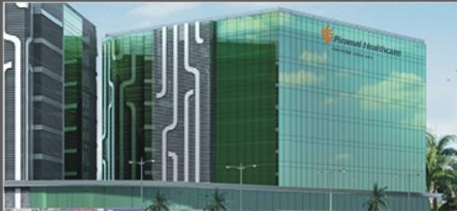
Piramal R & D Center, Mumbai Area: 100,000 ft 2 , HVAC Cost: Rs. 65,000,000
