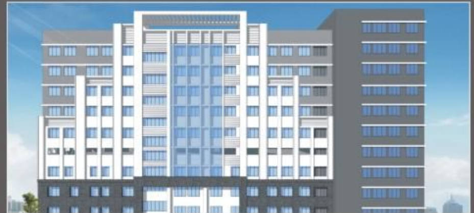
Bhabha Hospital, Bandra, Mumbai (IGBC Gold Building) 523 Beds , Area : 350,000 sq ft , MEP Cost : Rs. 780,000,000
