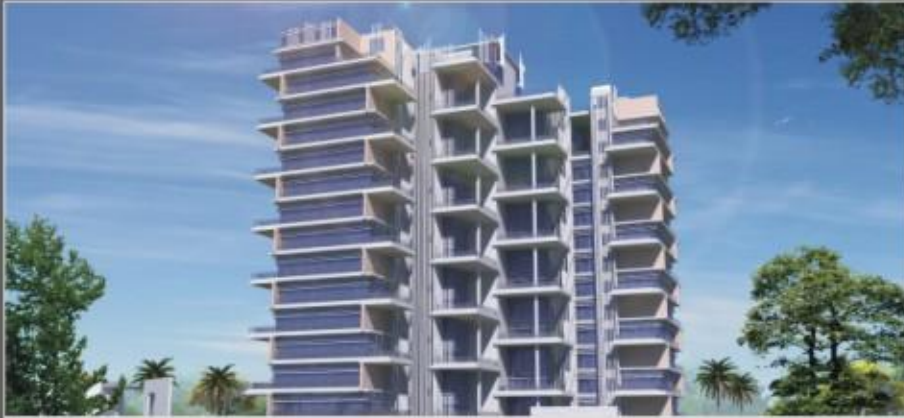
Ajmera High End Housing, Pune Area : 20,000 sq ft;Hvac: 600 TR VRV
