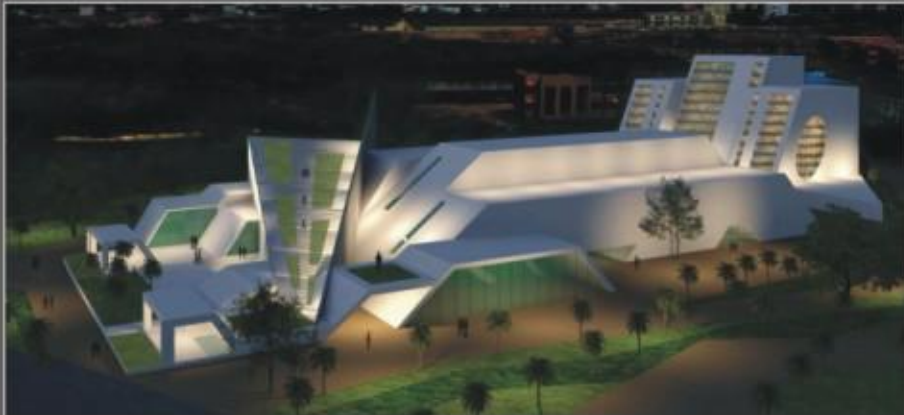
Tirupati International Convention Center Area – 120,000 ft 2 , HVAC – Rs. 72,000,000 – GRIHA Rated
