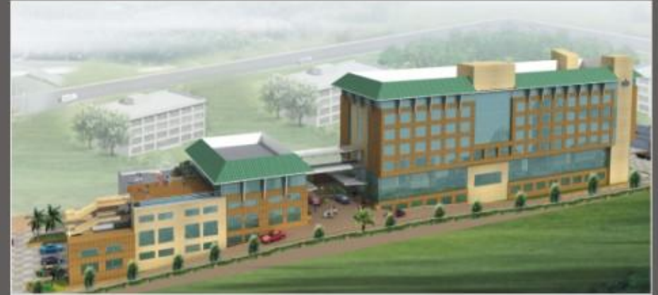
Country Inn & Suites (WHPL) Hinjewadi, Pune Area: 2,50,000sq ft, MEP cost: 120,000,000
