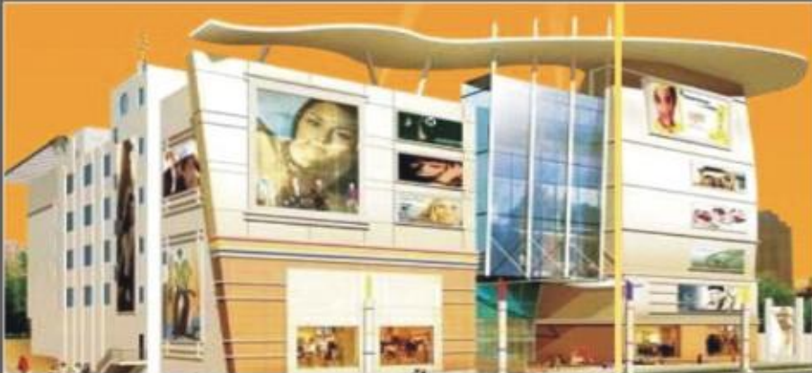
ASHOKA MALL AT HYDERABAD AREA:262000 SQ. FT.; HVAC:850 TR
